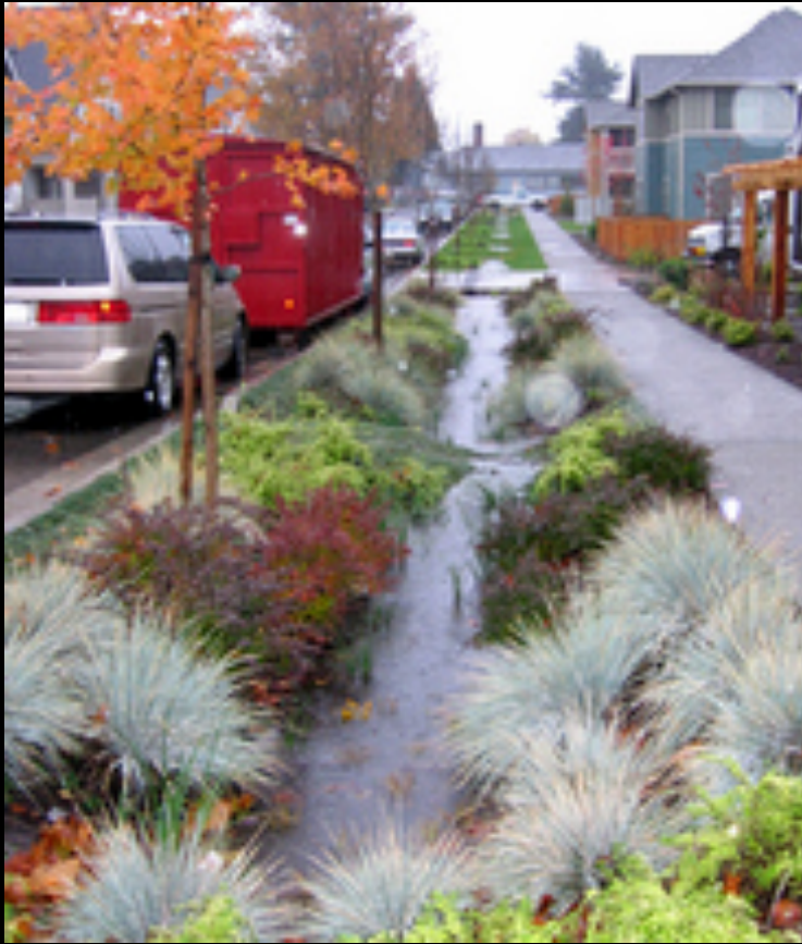
Stormwater captured with vegetated swales; U.S. EPA
